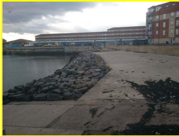
Revetment at north end of West harbour. (Asset ref. No. 1221C901C0401C23)
