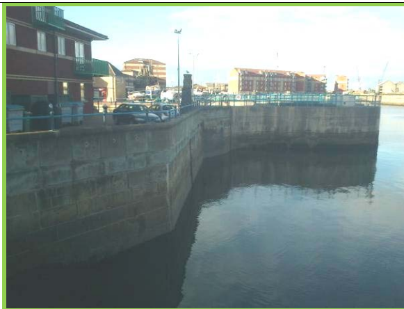
Wall to south side of lock entrance. (Asset ref. No. 1221C901C0401C25)
