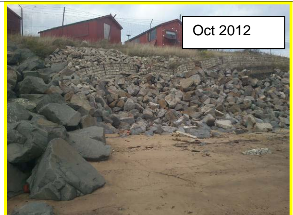
View of Gabion baskets with rock armour. (Asset ref. No. 1221C901C0401C17)
