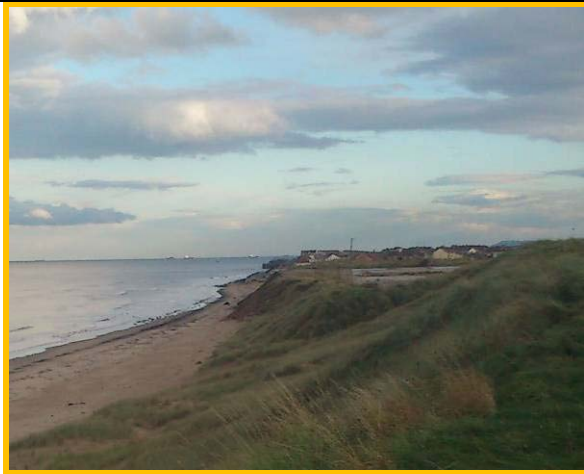
Eroding embankment east of cemetery in mid-distance (redevelopment underway). (Asset ref. No. 1221C901C0302C01)
