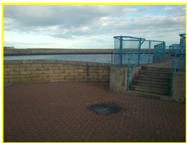
Flood wall tie into lock structure. Asset ref. No. 1221C901C0401C22)
