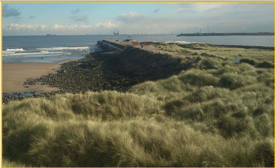
General view of North Gare breakwater. (Asset ref. No. 1221C901C0502C01)
