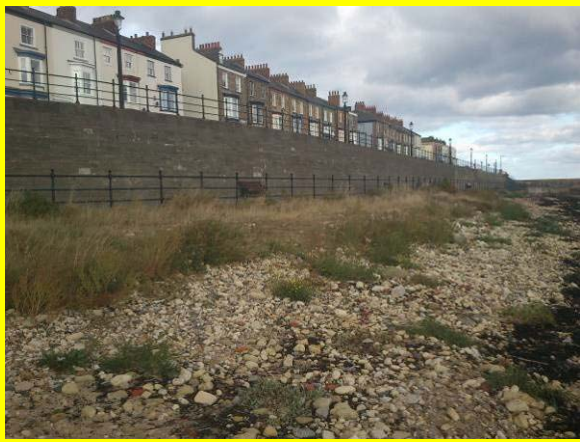
High cobble beach at mid-length of wall (Asset ref. No. 1221C901C0401C05)
