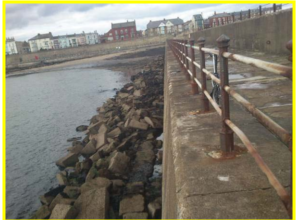
Armouring to toe of inner face of breakwater (Asset ref. No. 1221C901C0401C01)
