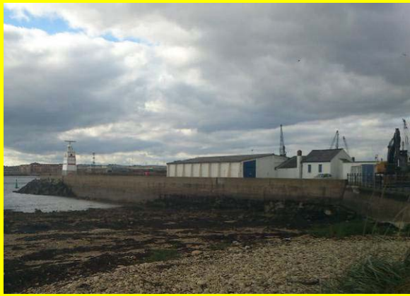
General view of Old Pier seaward side (Asset ref. No. 1221C901C0401C34)
