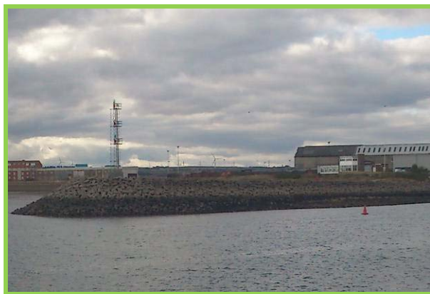
View of Accropode armoured breakwater. (Asset ref. No. 1221C901C0401C16)
