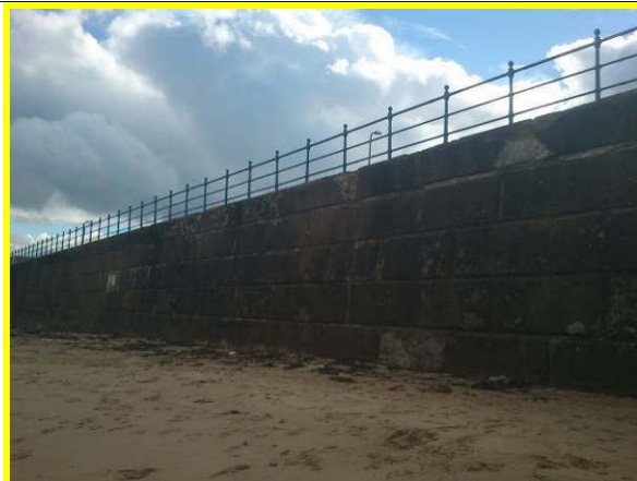
Blockwork wall at Sea View terrace. (Asset ref. No. 1221C901C0303C02)
