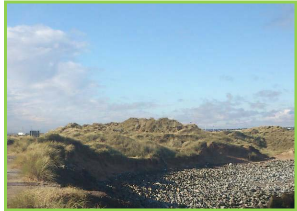
Localised cliffing of the dunes immediately north of North Gare, adjacent to rubble revetment placed to manage outflanking. (Asset ref. No. 1221C901C0502C01)
